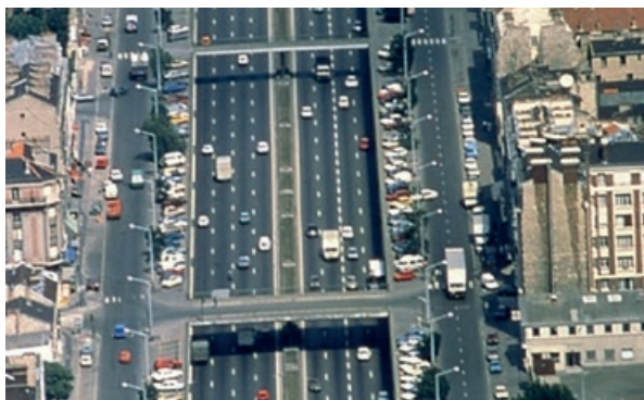
Photo 3 - Autoroute A1 avant requalification.
