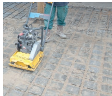
Photo 83 - Damage des joints.
